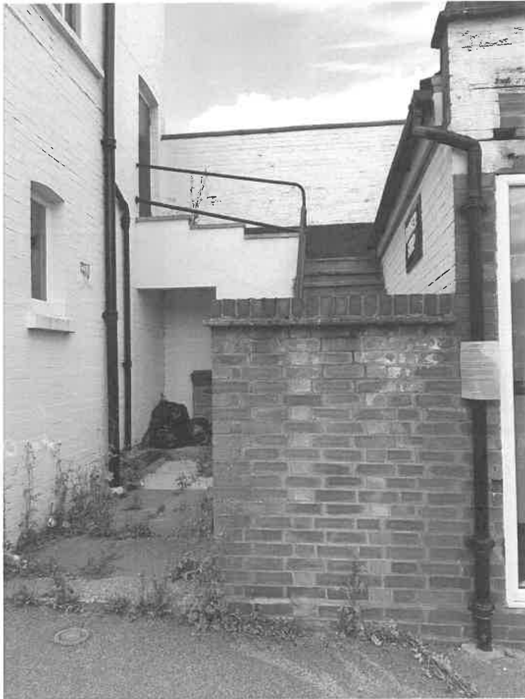
Photograph 7 showing adjacent yard proposed for smokers use
